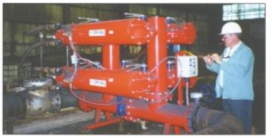
At 50 mic, the pre-assembled, Orival 46PEFL2 Filtration System, provides protection to the descaling pumps.
